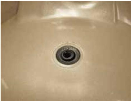
Tri-Valve (White) - Removable using a #2 Phillips head screwdriver
